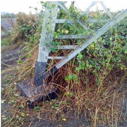
Image B.1 Photographs of L6 pylons showing steel lattice and foundation muffs
