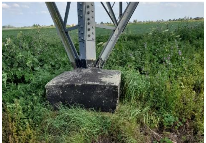
Image B.1 Photographs of L6 pylons showing steel lattice and foundation muffs
